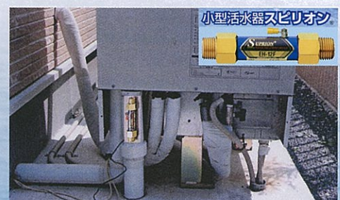
CO2 refrigerant applied Hot water boiler
